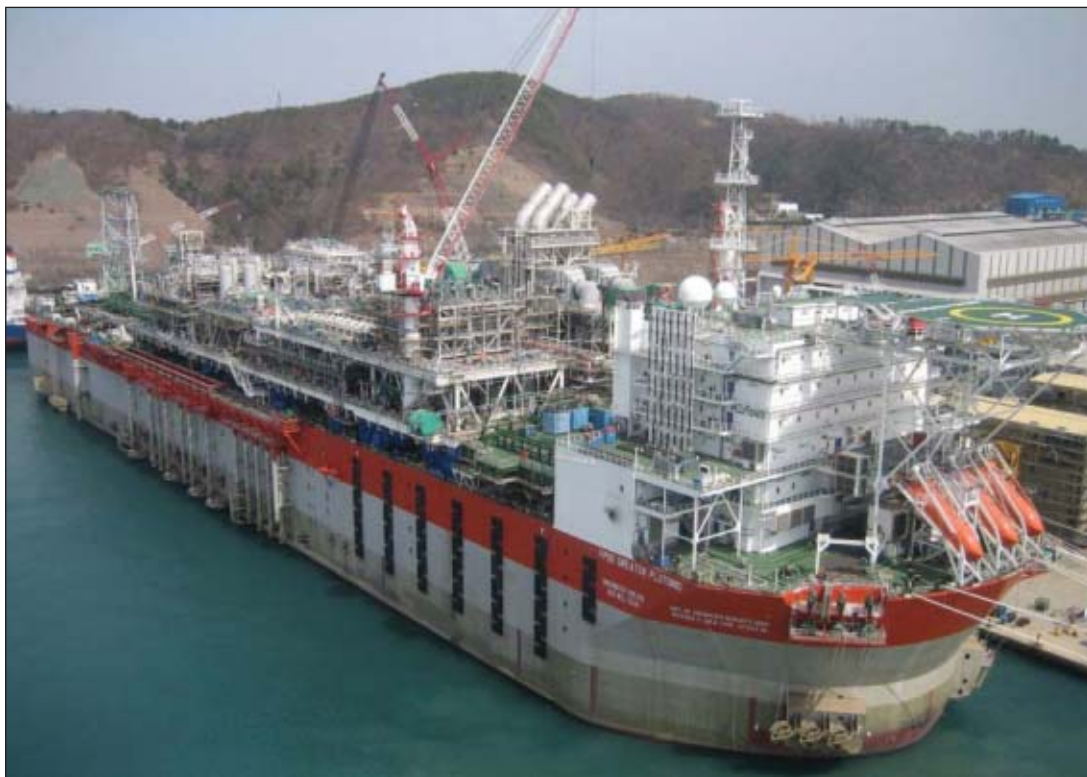
The floating production, storage, and offloading vessel for BP PLC’s Greater Plutonio complex off Angola, shown before tow-out, can store 1.77 million bbl of oil, process 240,000 b/d of oil, and handle 400 MMscfd of gas.
